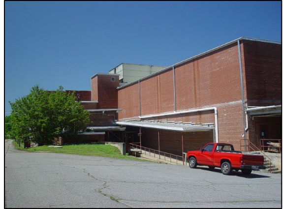
5. East side elevation (from rear of building)
