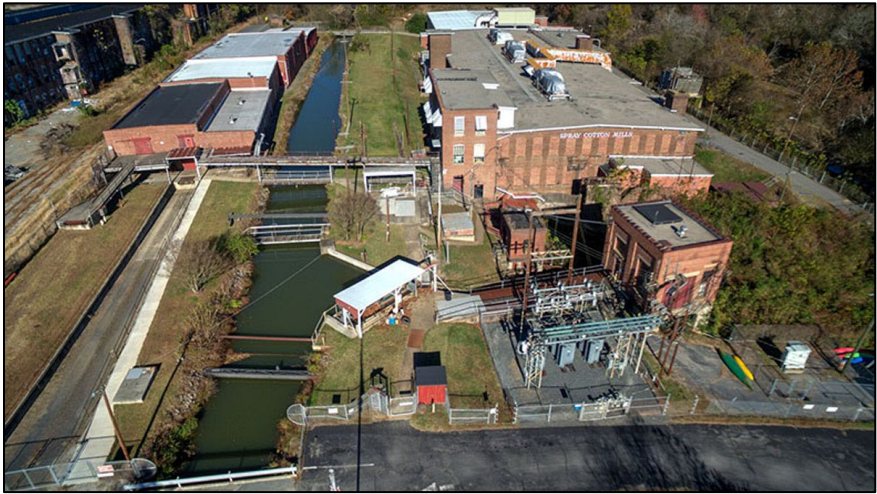
22. Overhead view showing main mill, power plant (lower) and power canal (left)
