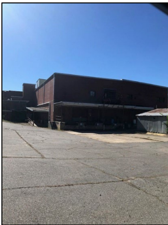
9. Rear elevation (later addition)
