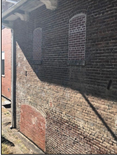
12. East side showing windows
