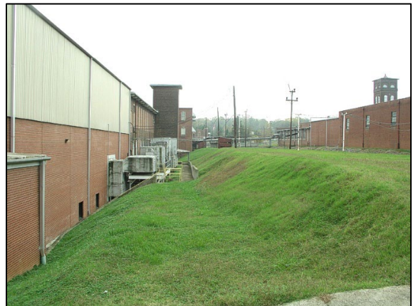
8. West side elevation (from rear of building)
