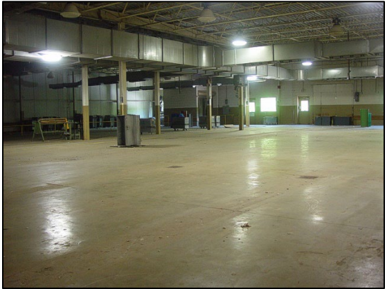
20. Interior of warehouse addition
