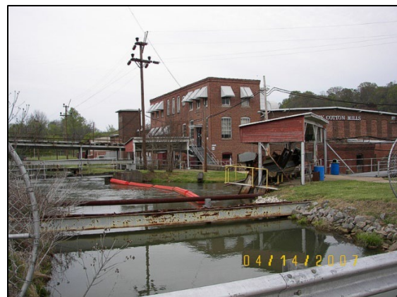
3. Southwest elevation showing office block
