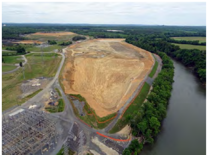
► Dan River ash basins after excavation (2019, via Duke Energy)
