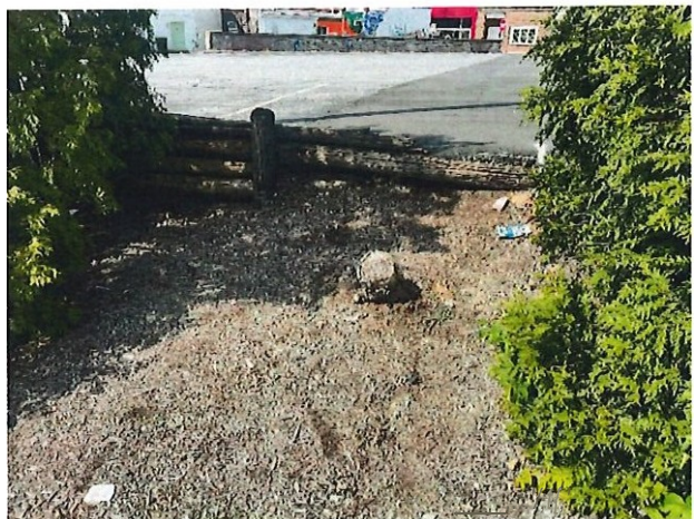
Figure 5: Retaining wall height varies along length.
