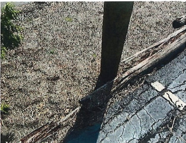
Figure 8: Active utility pole at base of retaining wall.
