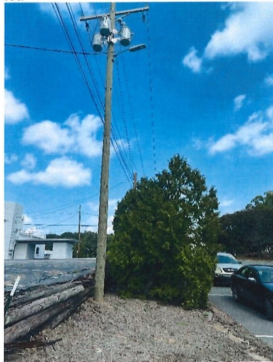
Figure 10: Utility poles located along length of retaining wall.
