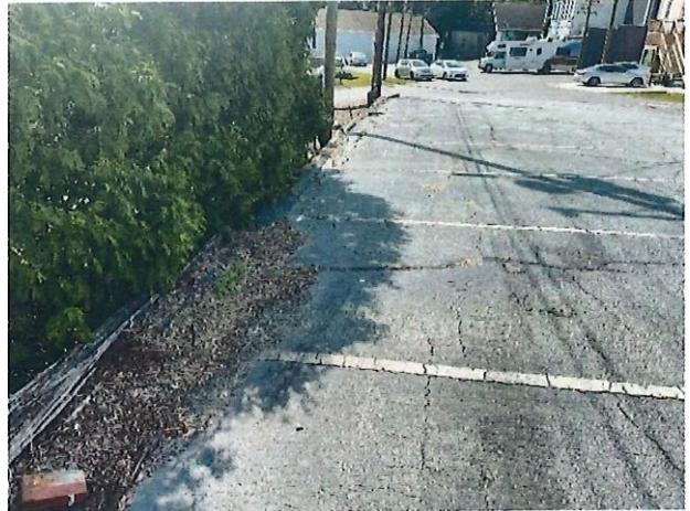
Figure 3: Upper parking lot looking southwest.
