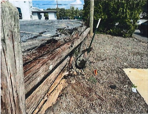
Figure 1 Looking northeast along the retaining wall, at high end.
